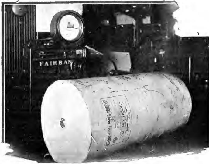
Weighing standard roll of news print paper on Fairbanks Dial Scales.
